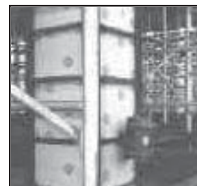
US-1600 with "Clamp-On" bracket on wooden form with steel reinforcing
